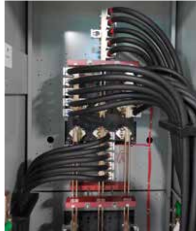
Automatic Transfer Switch
